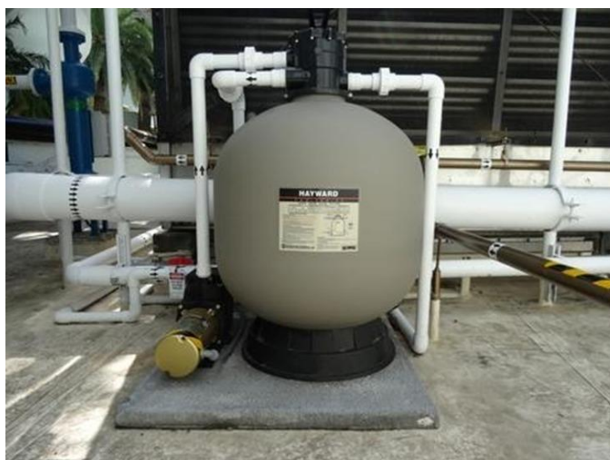
Example of Sewage Disposal
